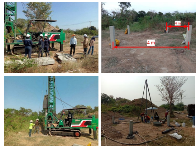
Figure 5. Precast PC 6 m. pile installation and soil survey.
