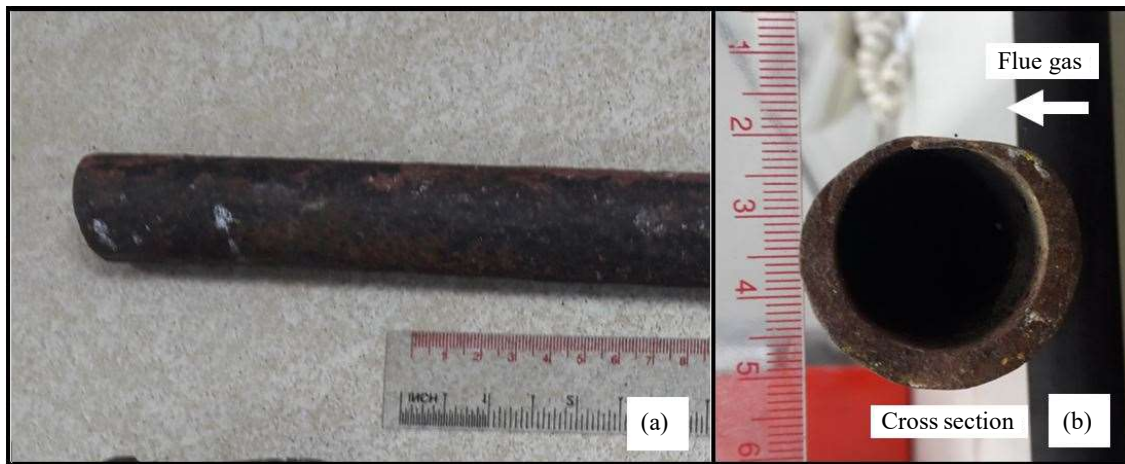
Figure 2. A sample cut from a failed superheat tube (a) overview, (b) cross section of tube.
